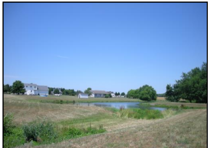
Stormwater Maintenance District Community Misty Pines
